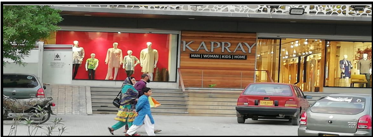
Fig. 2. The rise is found on an incorrect place and very vertical
