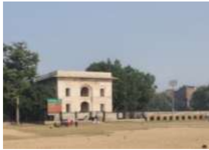
Figure 1: Tomb of Nadira Begum after conservation, showing causeway and houses on the backside
