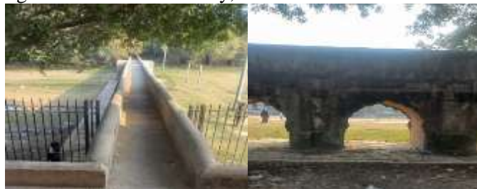
Figure 6 Side view of the causeway (Left) & Top view of the causeway (right)
